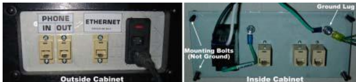
Figure 46. AC Power Plate (Standard Cabinet)
